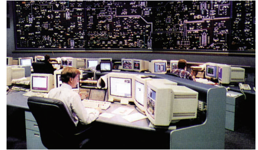
C++/Developer application displaying an entire transmission grid that monitors over 200 sub-stations and more than 120,000 SCADA points.
